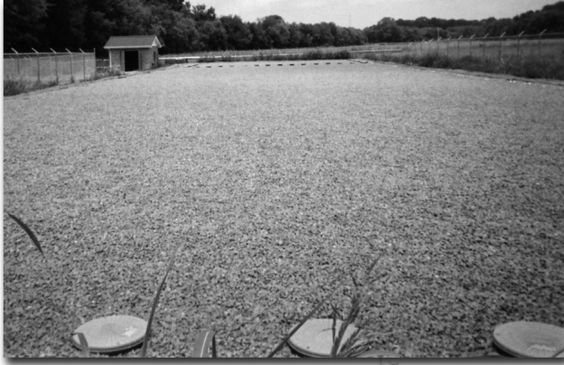
TENNESSEE 199 lot system - 60,000 GPD STEP collection system 55' x 217' recirculating gravel filter 10.4 acre - drip disposal field
