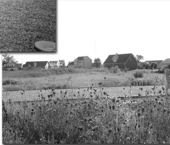
NORTHERN INDIANA 82 lot system 27,000 GPD STEP collection system 50' x 108' recirculating gravel filter
