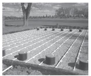
Zoeller Pump Company's Orifice Shields provide protection from the media or debris that surround an orifice in low pressure pipe applications. These simple, snap-on caps ensure that the flow from orifices in a lateral system remain uniform and consistent. Orifice shields are available in a solid cap for upward spray or a slotted cap for downward spray.
